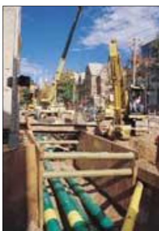
1 Construction on York Street, extending utility service from the Central Power Plant to the new School of Art
