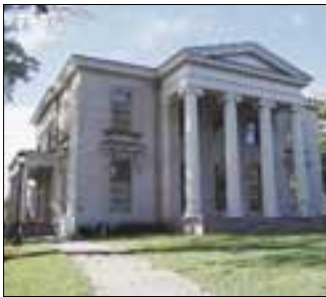
1 The recently restored 46 Hillhouse Avenue 2 Payne Whitney Gymnasium is an example of Yale’s historic heritage and is one of many locations for continuing University investment.
